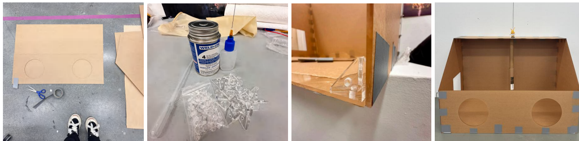
Fig. 11. Assembly process of the laboratory glove box. From left to right: (1) Cut acrylic sheets prepared for construction, (2) Weld-On #4 acrylic adhesive and transparent acrylic corner bracket, (3) Drilled and fixed transparent acrylic corner bracket, (4) Assembled structure left to dry.
