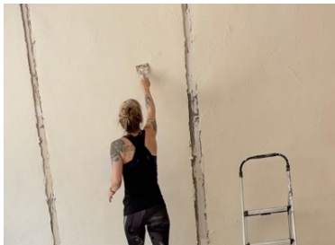
Figure A.5b. Intonaco Surface Prep
