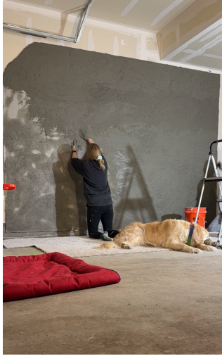
Figure A.5. Fresco Base Layer Application (Step 1)
